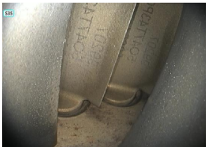
STAGE 5 CORROSION/PITTING INDICATION EXAMPLE
