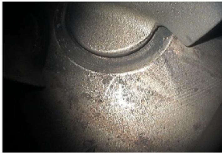
STAGE 5 CORROSION/PITTING INDICATION EXAMPLE
