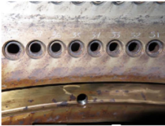
DISASSEMBLY CONDITIONS SHOWING CORROSION/PITTING OXIDATION FINDINGS (STAGE 5 AND STAGE 6)
